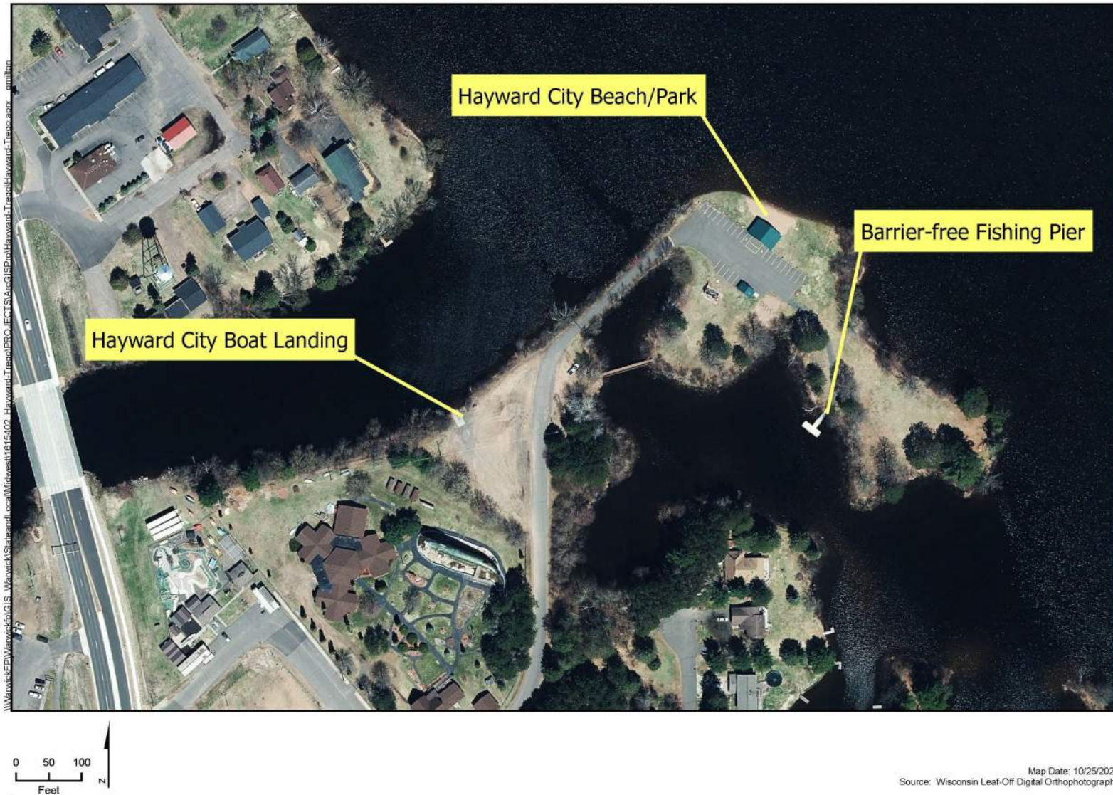
Figure 3-2. Hayward Project Recreation Facilities – Upstream Areas.
